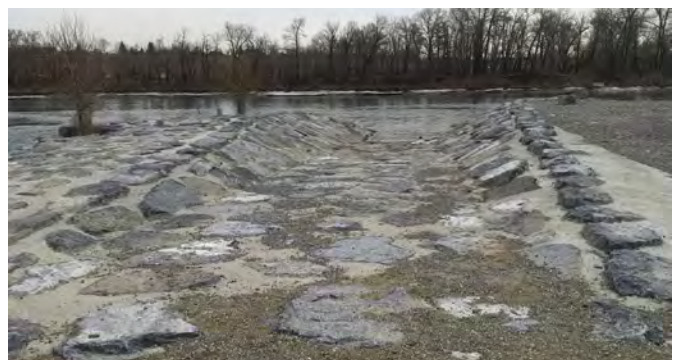
HARVIE PASSAGE LIMITED ACCESS BOAT RAMP
