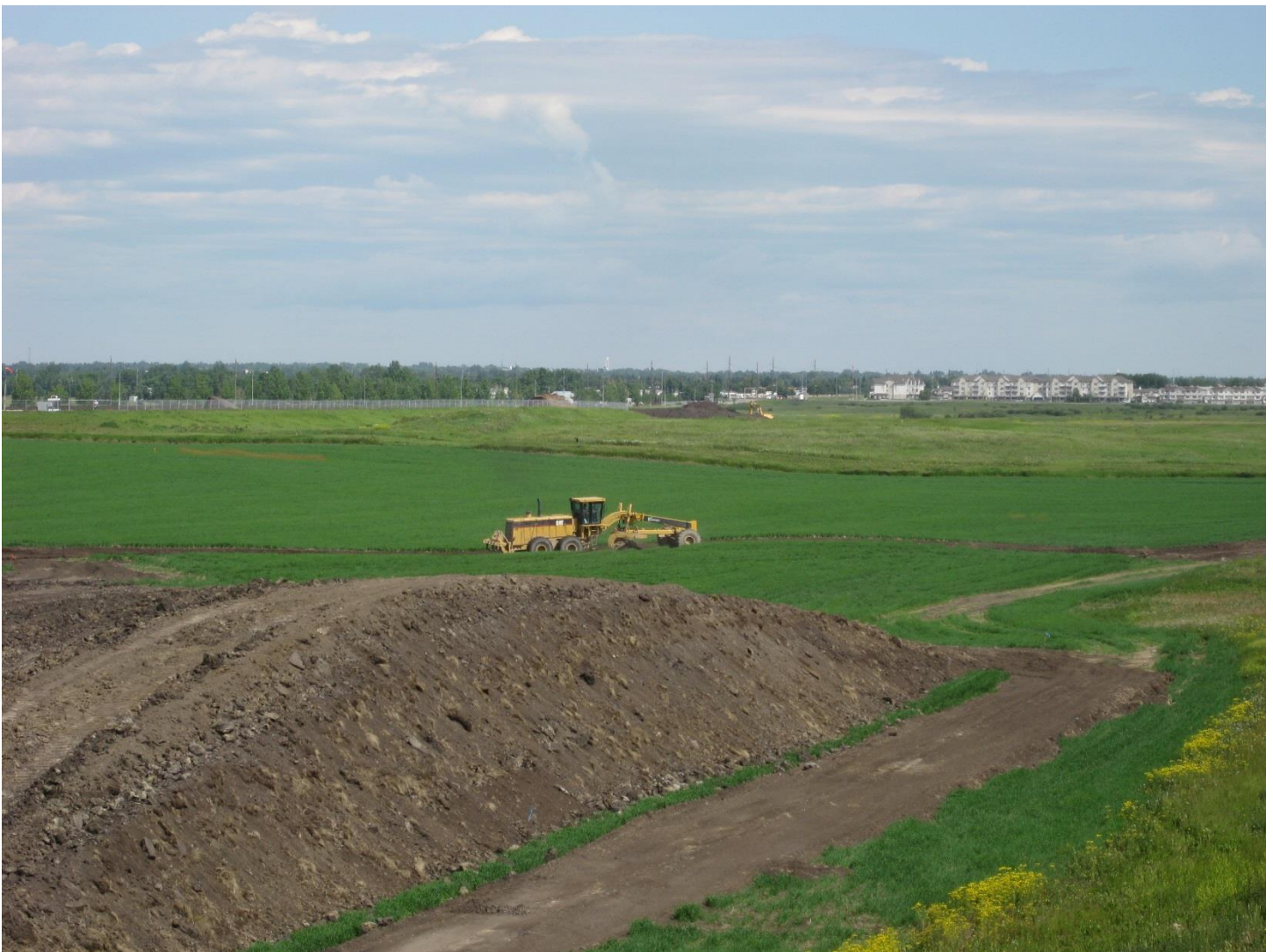
Proper soil handling practices shown through minimizing stockpile depth and clearly delineating access routes.
