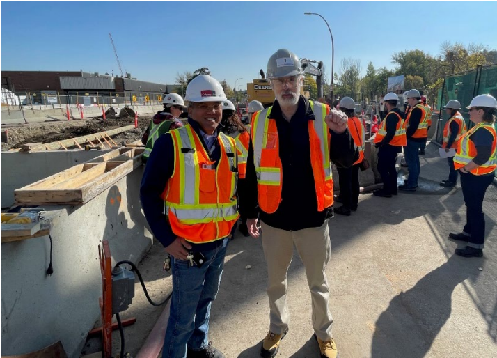
Councillor Pootmans and Councillor Wong visited the Beltline East utility relocation project site on September 12 with representatives from Alberta Roadbuilders and Heavy Construction Association.
