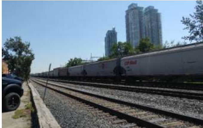
Figure 3.4: CP mainline through Calgary showing residential developments in the background
