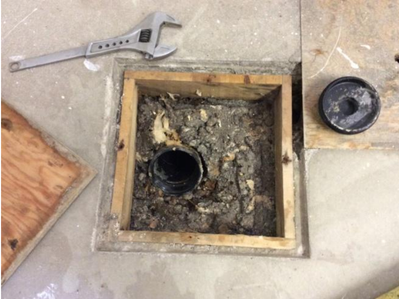
Figure 1 Cleanout in the floor
