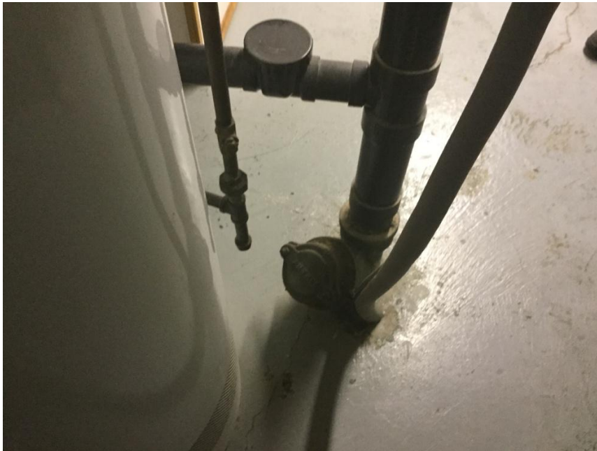
Figure 5: Sometimes this type of stack can be used, but in the interest of protecting your property from damage Water Services crews prefer to work from the cleanout.
