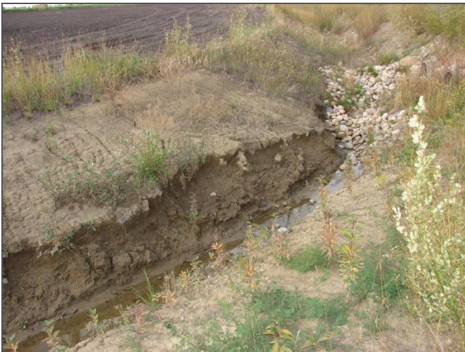
Photo 8 Channel Erosion
