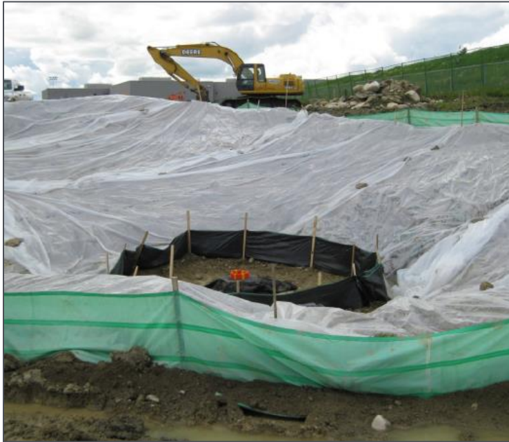
Photo 3 Isolation Measures, Poly Sheeting
