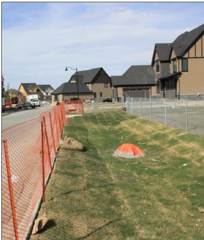
Photo 4 Temporary Sod Cover
