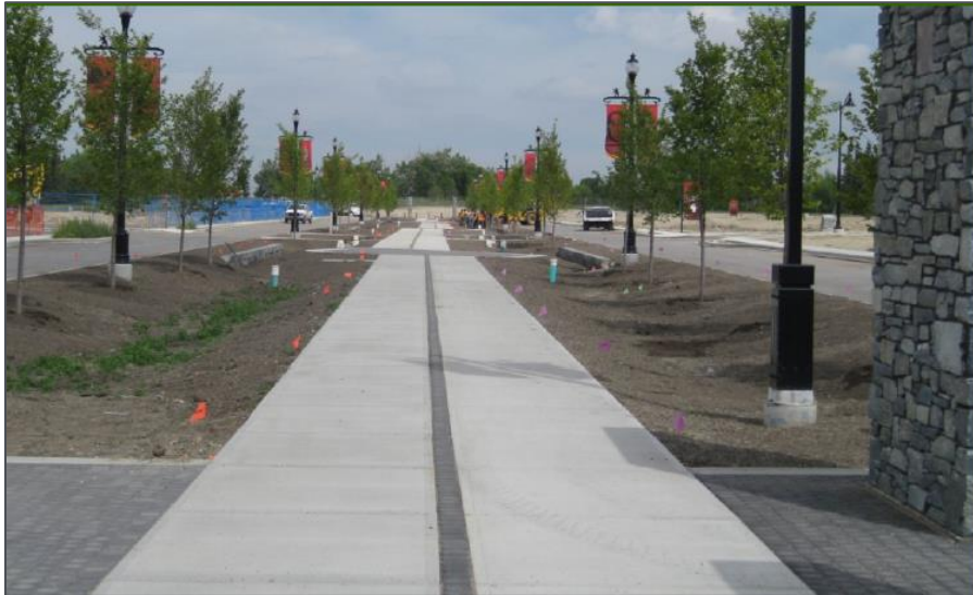
Photo 2 Installing Low-impact Developments Last is the Preferred Construction Method
