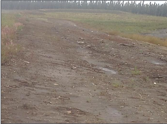
Photo 5 Sheet Erosion
