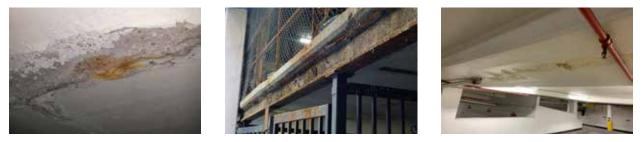
Damaged or Debonded Expansion Joints / Debonded Traffic Deck
