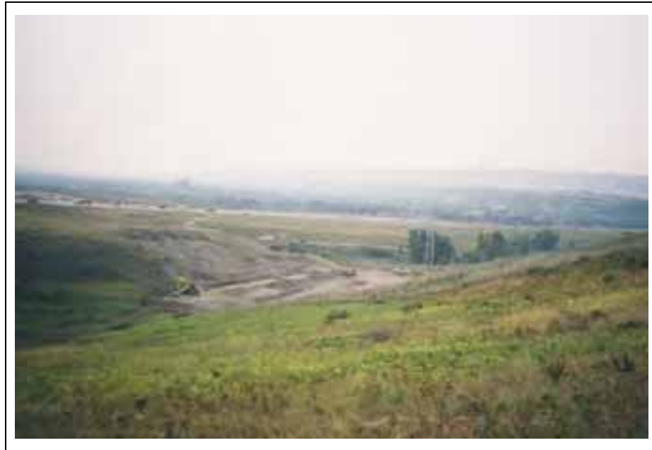
Photo 11: Road development across drainage.
