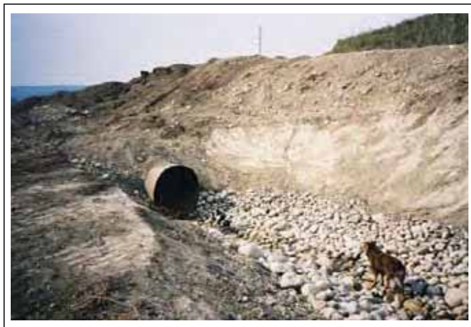
Photo 12: Culvert system for maintaining creek flow during road construction.
