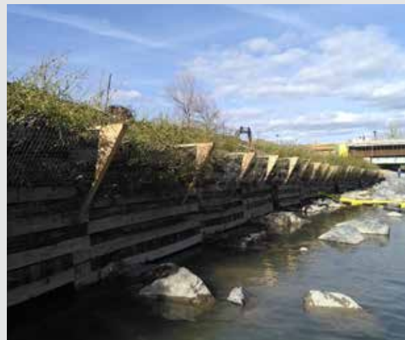
Before (left) and after (right) at the BDEP – a new bioengineering timber crib wall and boulders placed in the river create improved fish habitat, enhance bank stabilization and improve biodiversity.
