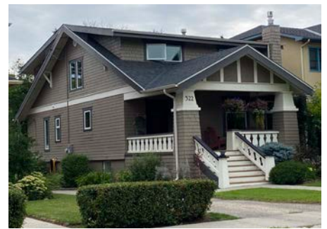
Compound roof pitches
