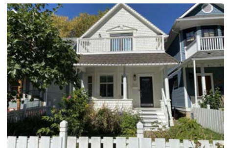
Example of deck projecting above the main floor
