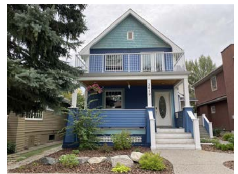
Example of deck projecting above the main floor
