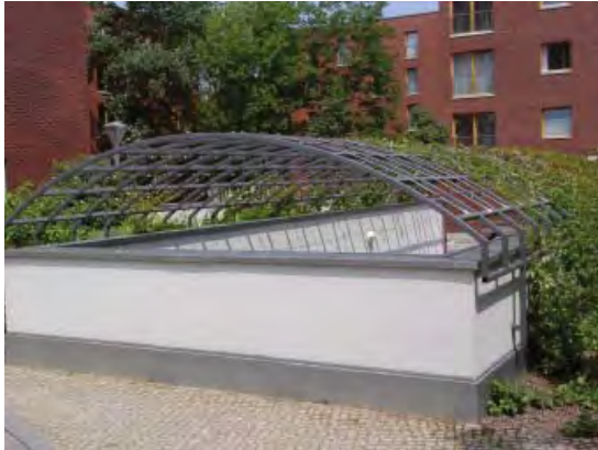
Entrance to a residential underground parkade
