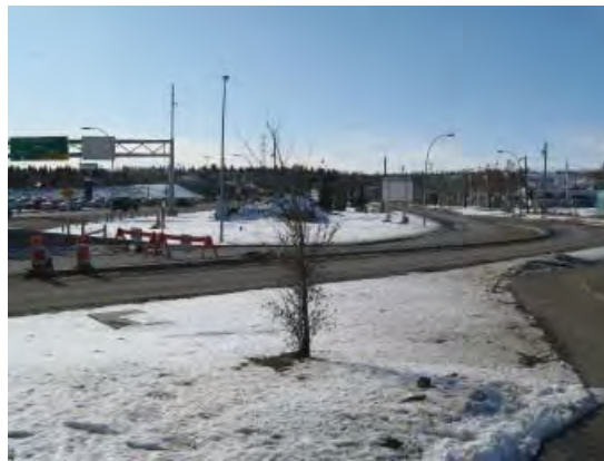
Bow Trail looking west
