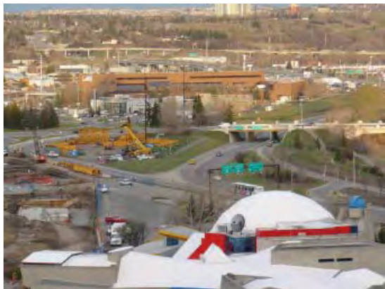
14th Street S.W. bridge and junction
