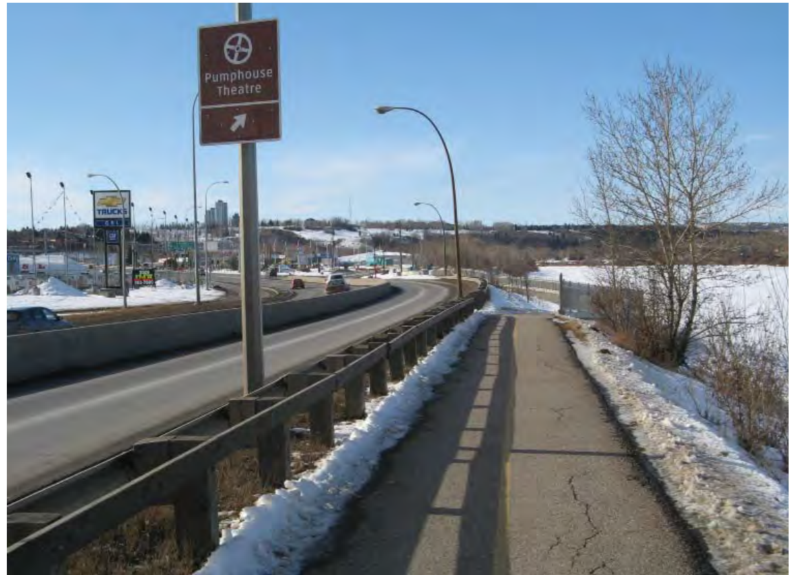
Existing situation along the Bow River
