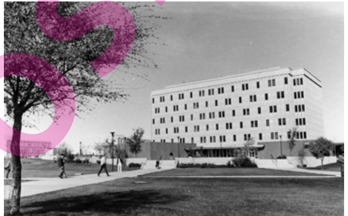
Photo: "University of Calgary Science Building, Calgary, Alberta." 1970, by Fred Kobsted. City of Calgary Archives, CaIA PP-01452.
