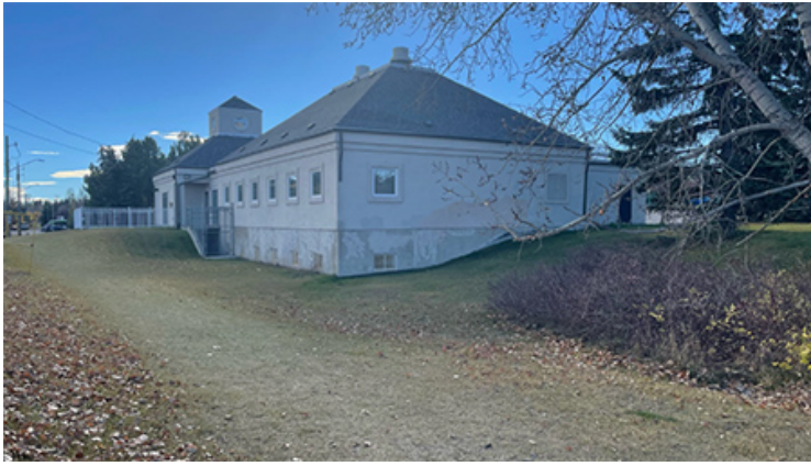
Exterior view from NE looking SW
