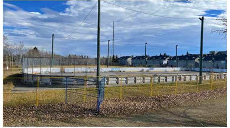
Exterior - rink (surrounding boards to be demolished)
