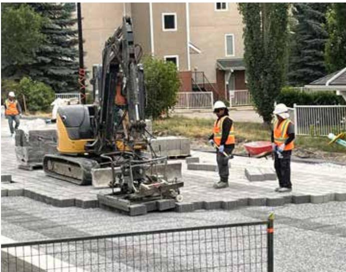
Marda Loop permeable pavement installation
