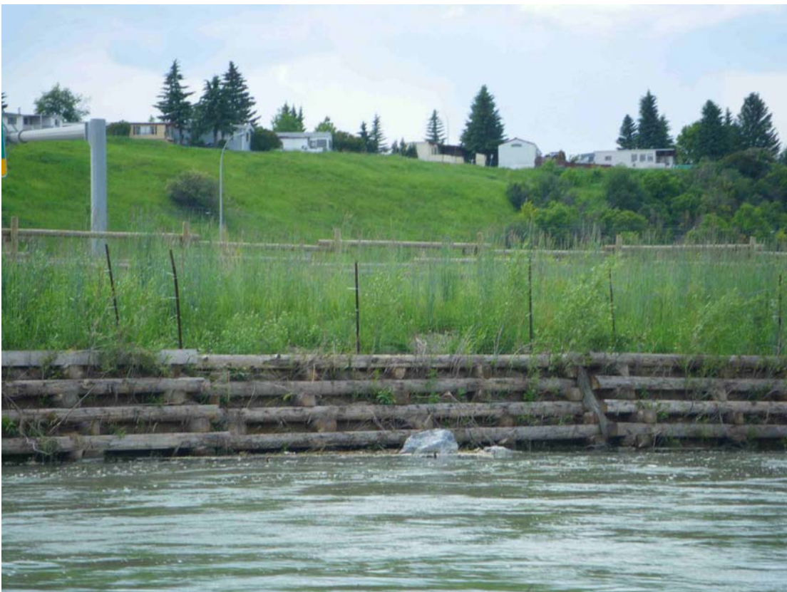
Figure 12. Live Crib Wall along Bow River, near Deerfoot Meadows, South Calgary
