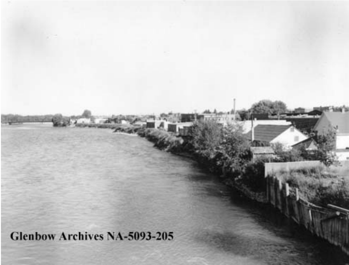
Figure 14. South Bank of Bow River viewed from Centre St. bridge, Calgary, AB
