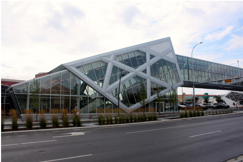
Figure 7 | 61 Avenue SW Pedestrian Bridge
