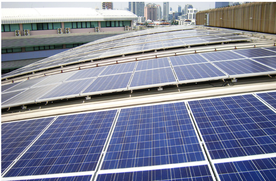
Figure 20 | Solar panels on an industrial building
